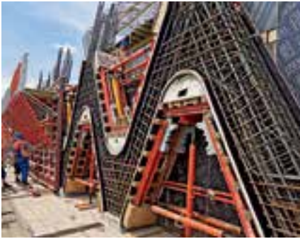
Prosta Tower, Warsaw, Poland
