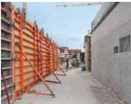
TRIO Structure is a variant of the proven panel formwork system and can be used with the complete range of TRIO accessories.
