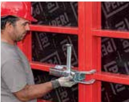
The BFD Alignment Coupler can be operated using one hand only.
